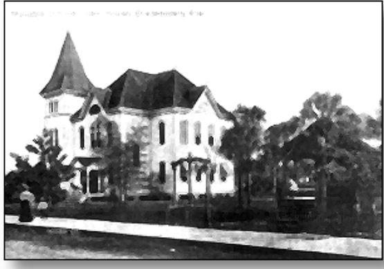
Manatee County Courthouse, Courthouse Square, Bradenton, c. 1900.
